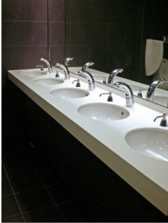
water tap c/w infrared sensor
