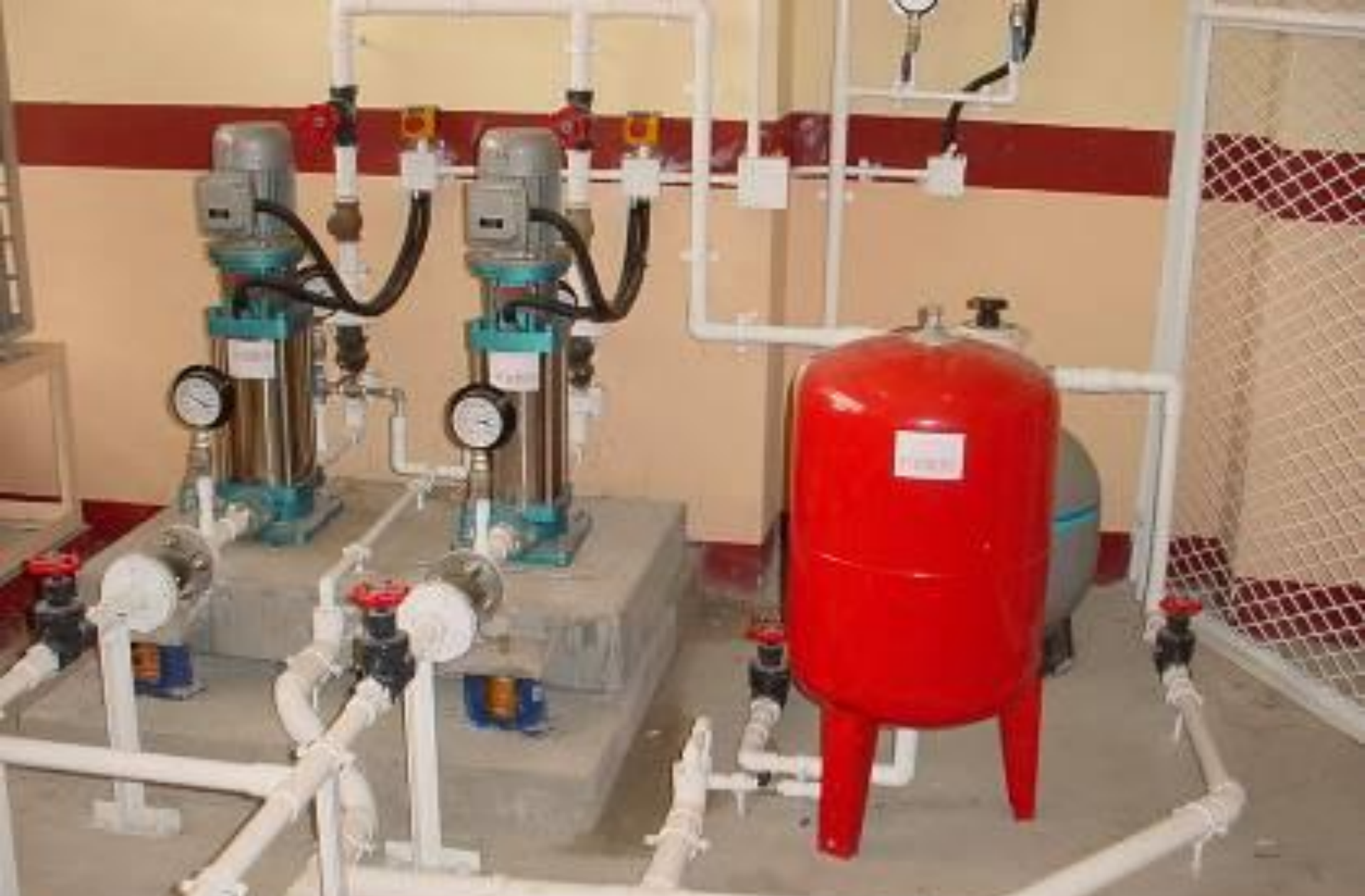
Rainwater Harvesting System
