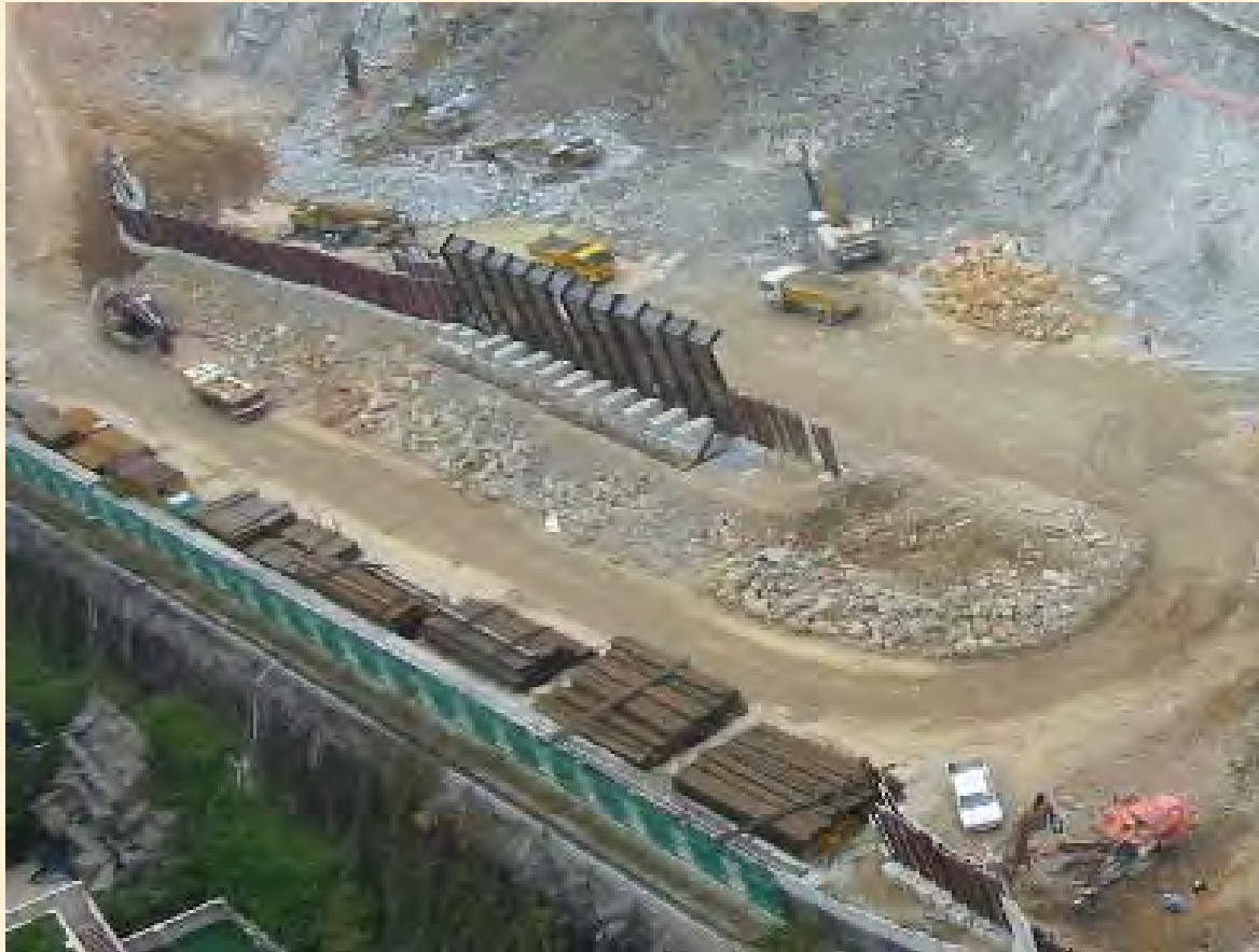
Noise Barrier (Road T7)
