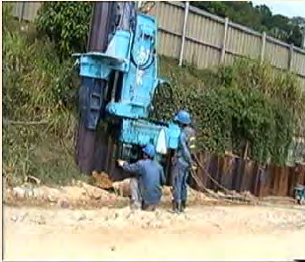
Silent Piler for Sheet Piling (MOS Rail)
