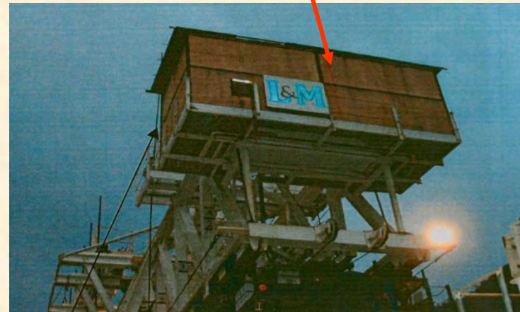
Noise Enclosure for Engines (Road T7)
